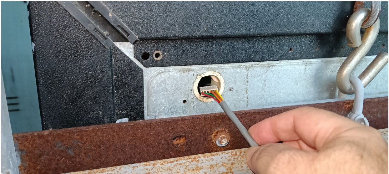
Pull through the cable slack
